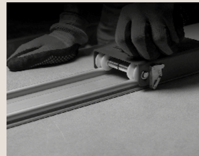
Cutting detail with guide on slab
